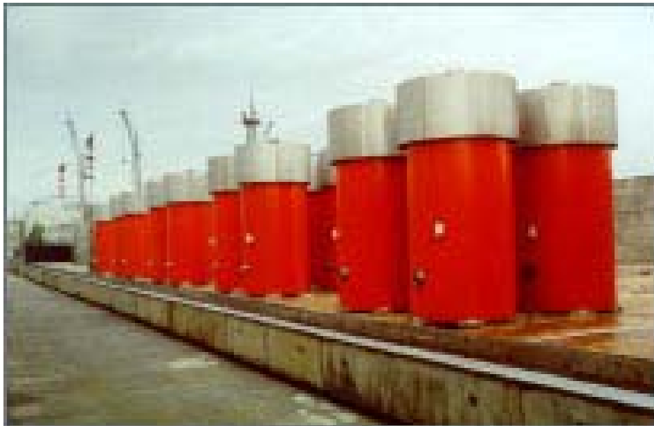
Fig. 5. Containers of the spent nuclear fuel storage
