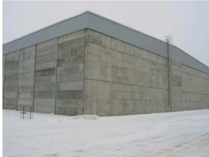
Figure 2.2.5-1. Partial view of building 158/2.
