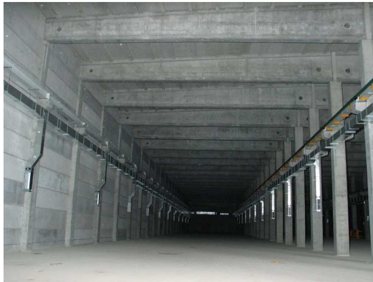
Figure 2.2.5-2. Partial inside view of the building 158/2
