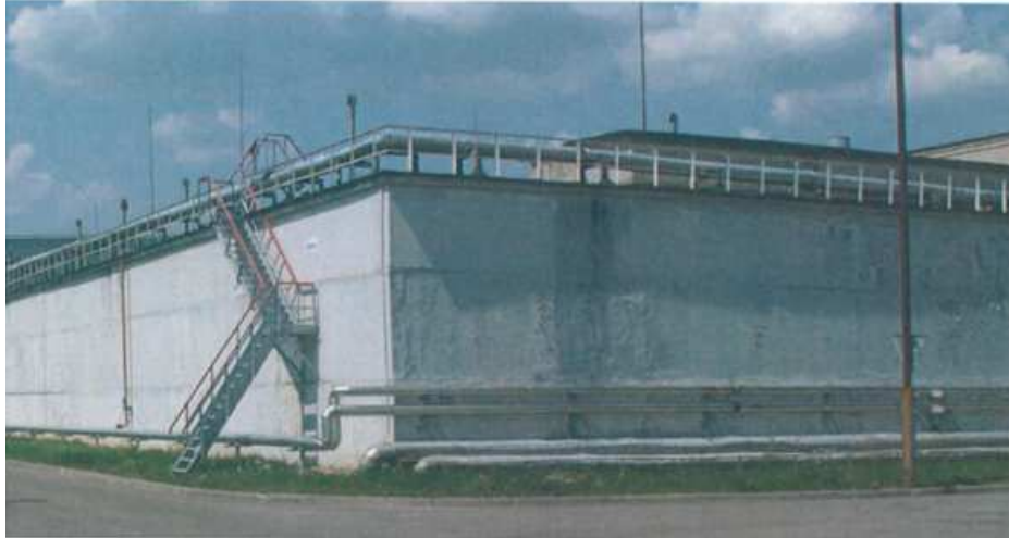
Figure 2.2.4-1. Partial view of the Bituminized Radioactive Waste Storage Facility
